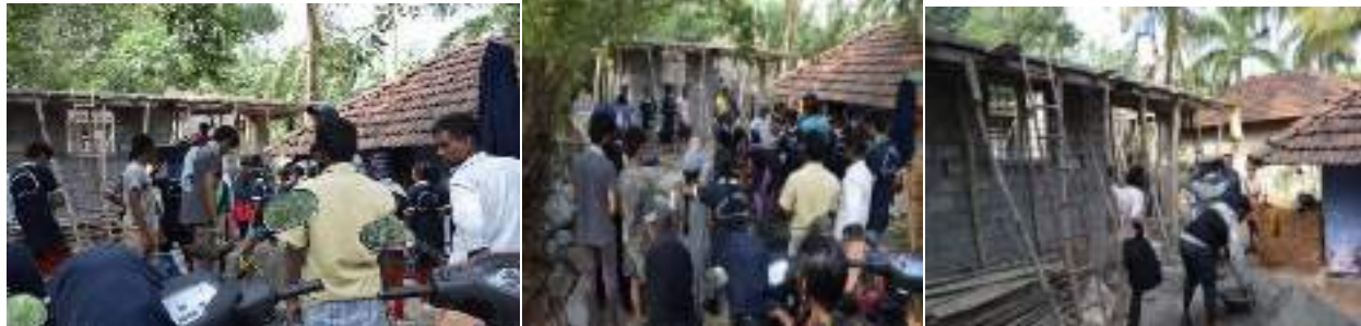
ABHAYAM-HOME FOR HOMELESS – SUNSHIDE CONCRETING
